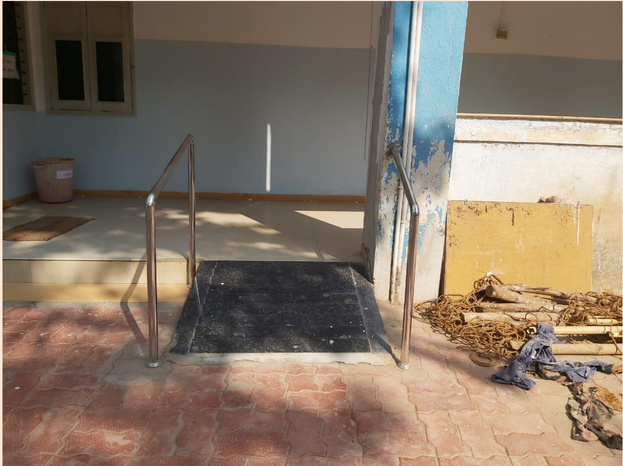
A Wheelchair Ramp on North Side of the College-To Move Freely and Safely
