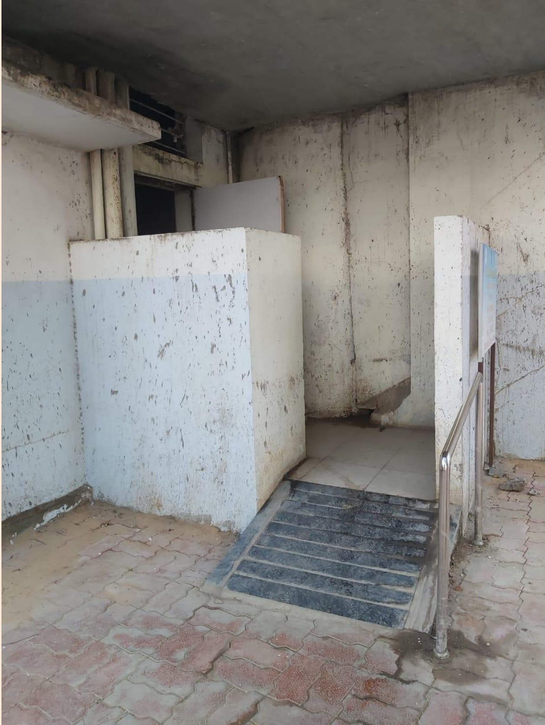
A Wheelchair Ramp at the Entrance of the Washroom
